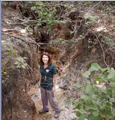
BANK STABILIZATION OF HEADCUT IN SIDE CHANNEL TO MAIN STEM AT CHESAPEAKE COLLEGE, BEFORE AND AFTER RESTORATION - APPROX 8 FT DEEP 5 FT WIDE
