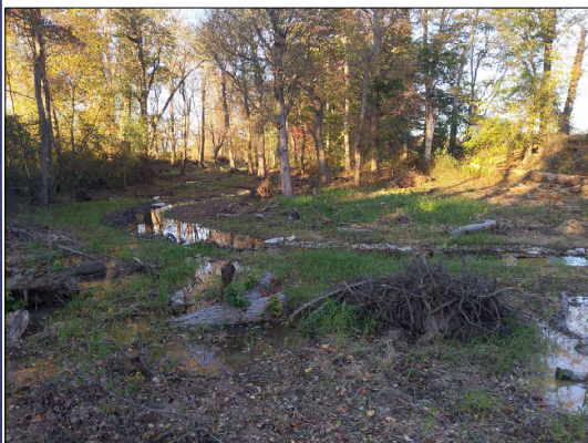
RECONSTRUCTED STREAM BED IS ELEVATED AND REDUCED TO FORCE WATER ONTO THE FLOODPLAIN AND SLOW IT DOWN
