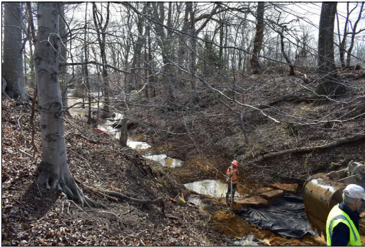
EXAMPLE OF BANK STABILIZATION TO A HEADCUT RAVINE AT KING'S CREEK TALBOT COUNTY MD
