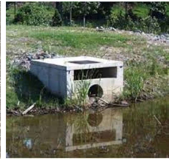
C EXAMPLE OUTLET STRUCTURE
